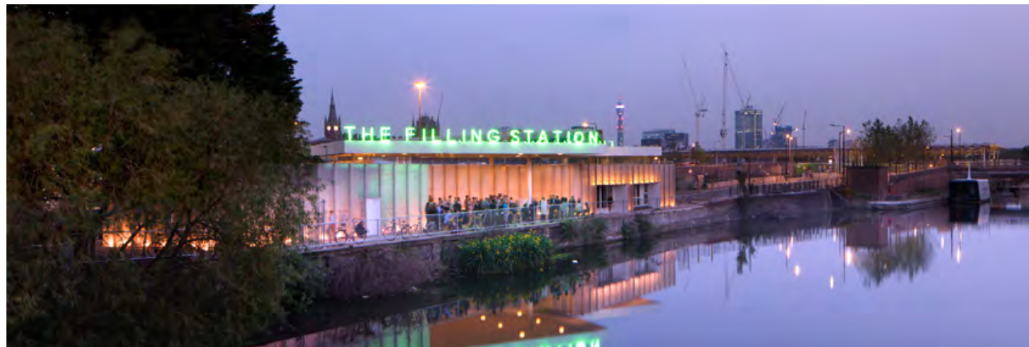
“The Filling Station,” designed by Carmody Groarke, was a derelict gas station converted into an impermanent public-events space and restaurant. Using the existing canopy and forecourt, the space was enclosed by a prefabricated fiberglass screen. Photo courtesy of Carmody Groarke
